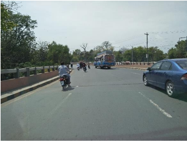
Figure 2-15: Abdullah Pur Overpass
