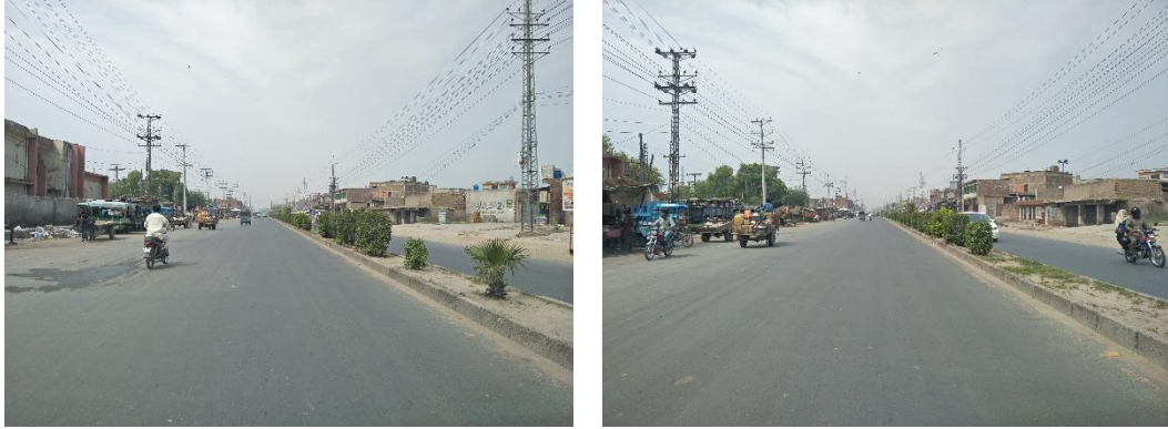
Figure 2-4: Existing Features of Sheikhupura Road
