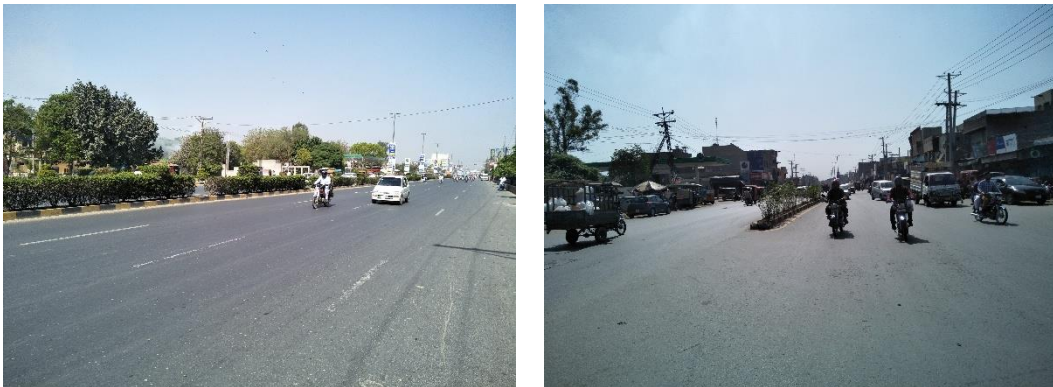
Figure 2-5: Existing Features of Jaranwala Road
