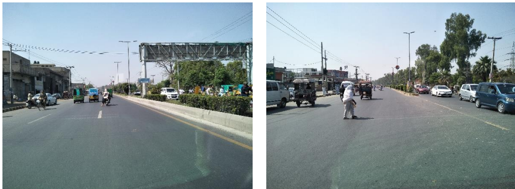
Figure 2-7: Existing Features of Sammundari Road
